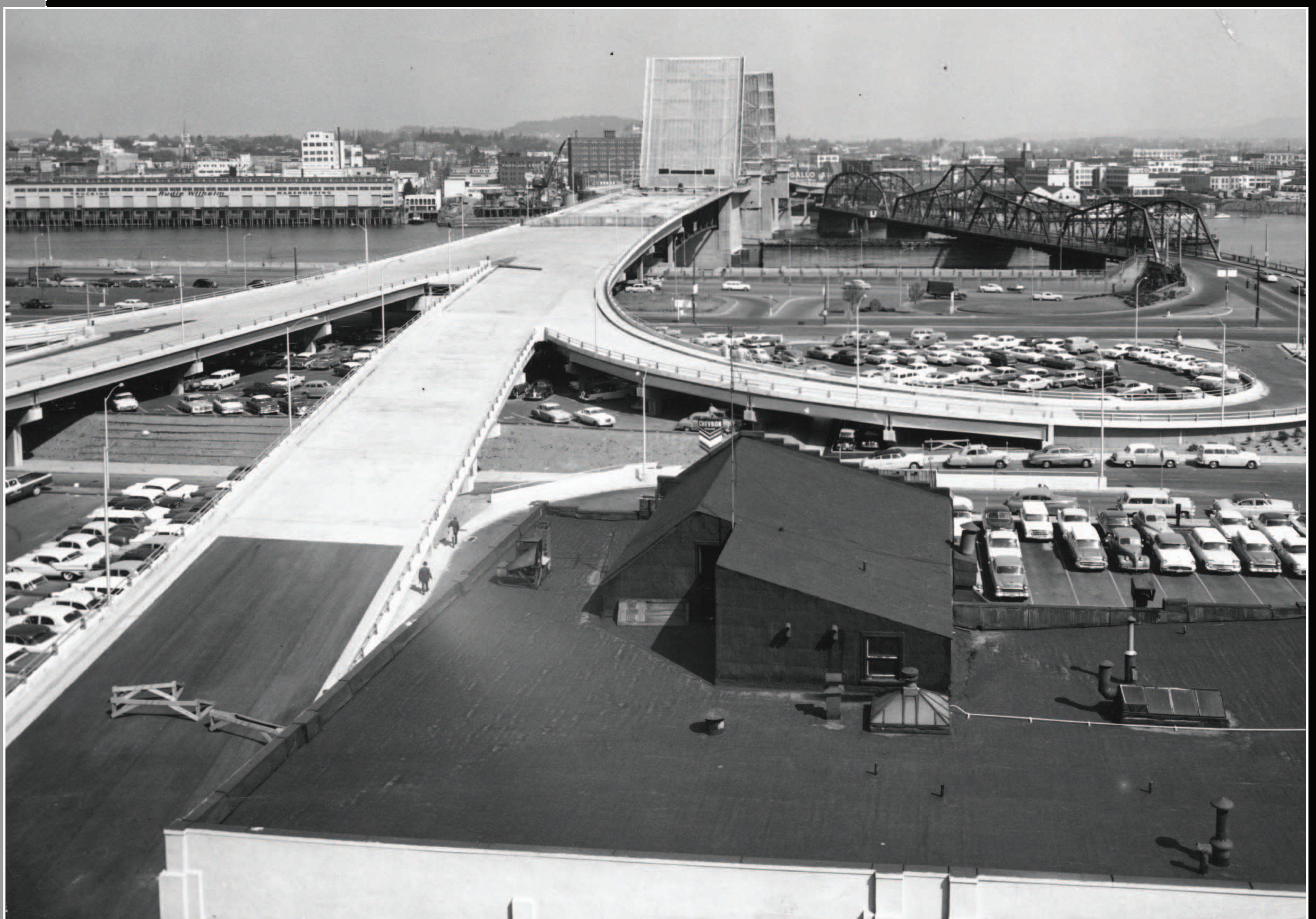
CONSTRUCTION OF THE NEW MORRISON BRIDGE, 1958
