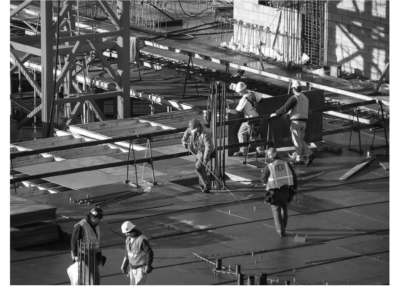
Cherry City Electric on the job.
