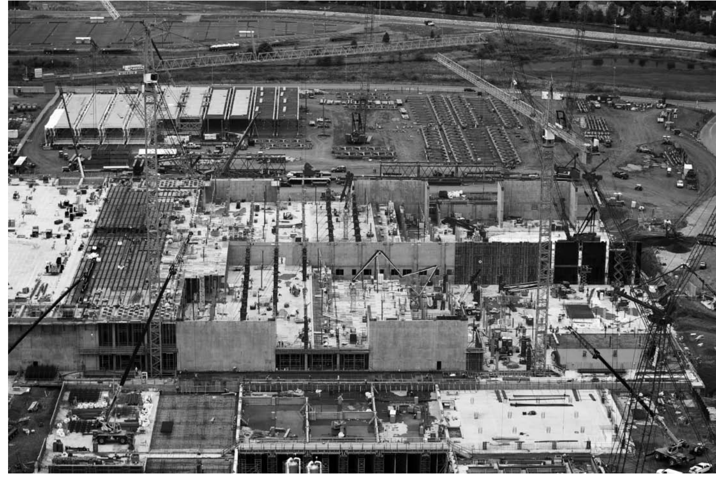
Construction of Intel's DX1 fabrication facility in Hillsboro, OR.
