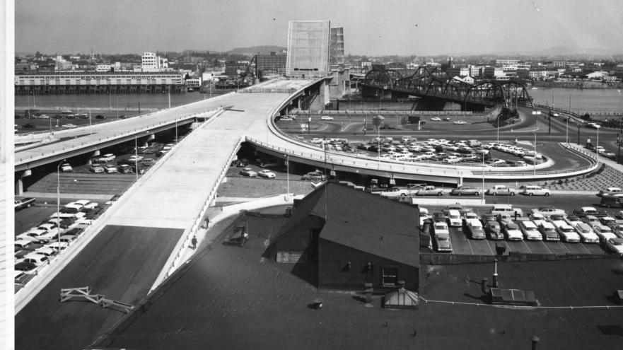
Wired and just about ready for electric traffic gates, the new Morrison Bridge, with its double-leaf bascule spans raised nearly vertical in this 1958 photo, contrasted sharply with the old Morrison Bridge, built in 1905, that it would replace.
