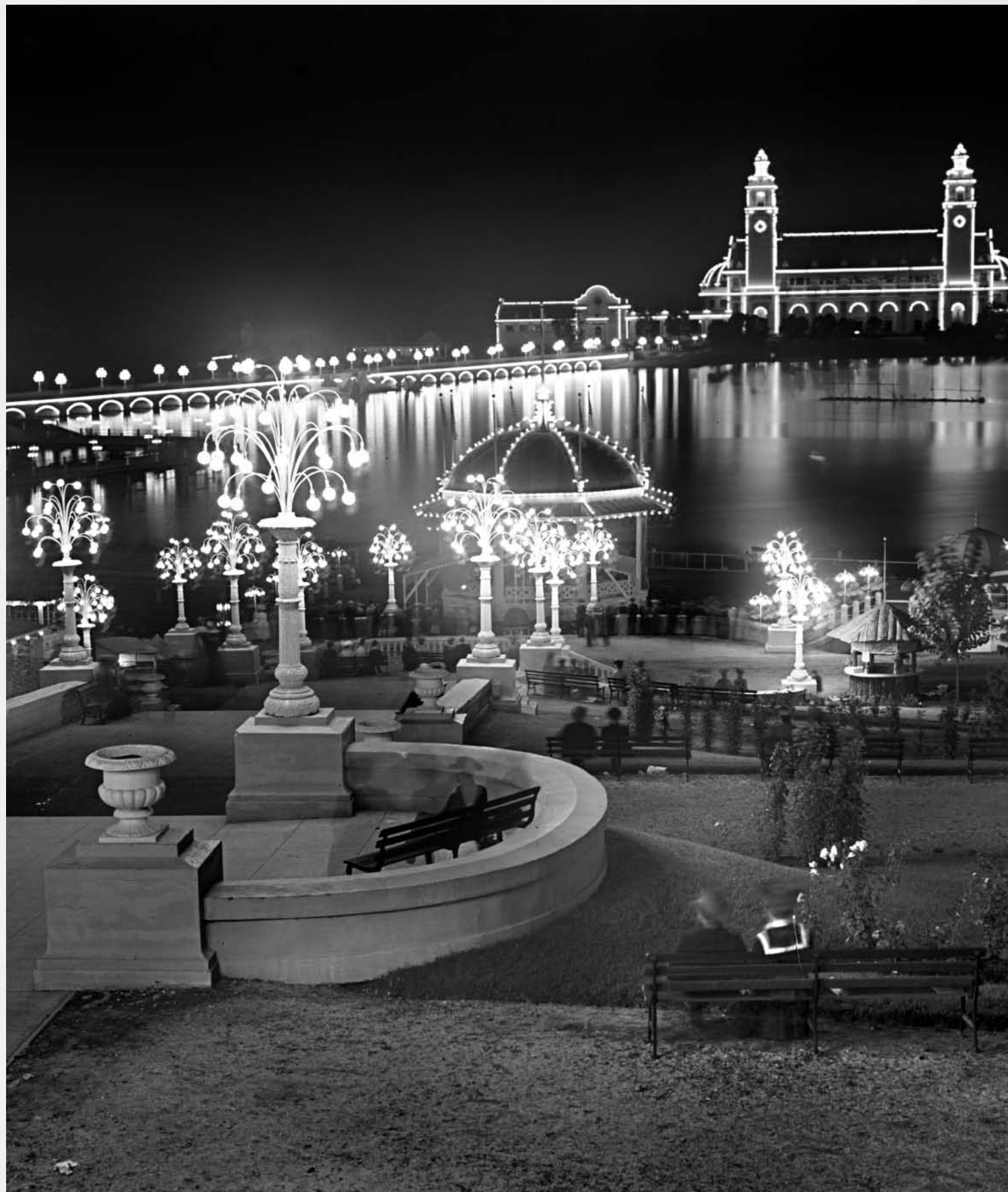
The electroliers (electric chandeliers) that lit Guild's Lake and outlined the Lewis and Clark Exposition demonstrated the skill and necessity of a new industry, that of the electrical contractor and his electricians.
